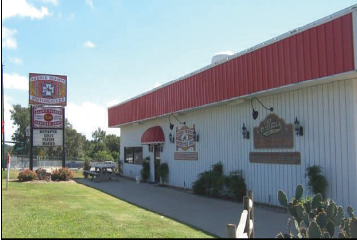
Sign & Front of Bldg. #1 on US 441
