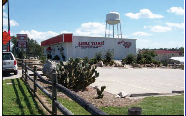
West Side of Bldg. #1 on US 441
